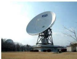
KDD Ibaraki Satellite Communication Center
